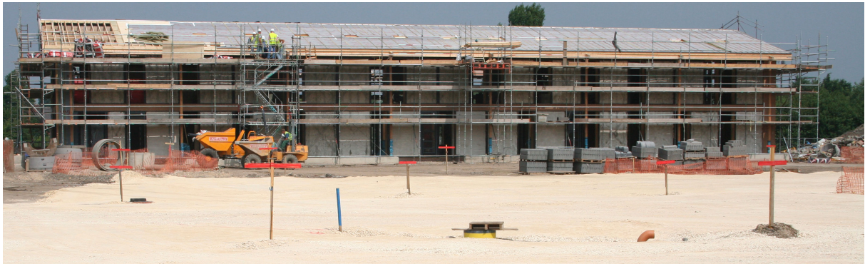
Work on York's Eco-depot October 2006 © Christian Vassie
